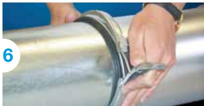
6 Snap QF clip over the O-ring and one end of the slip duct
