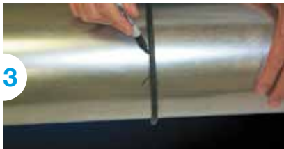
3 Use O-ring provided and mark for cut.
