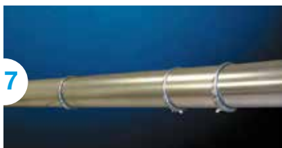
7 Finished connection with the slip duct.
